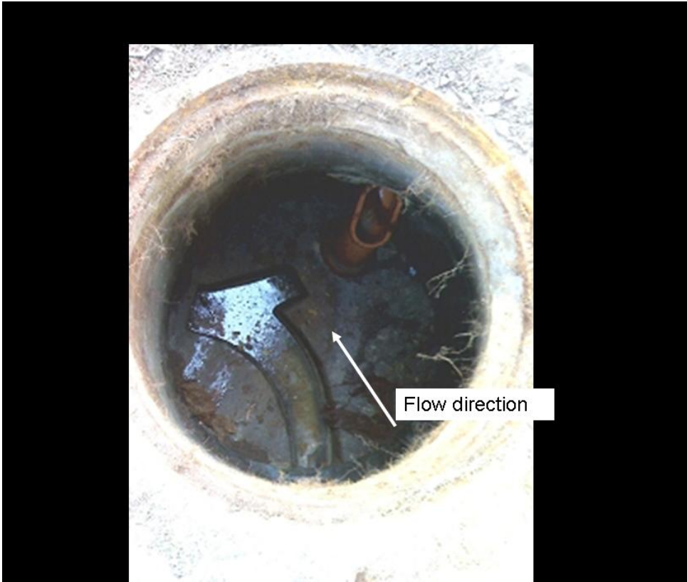
Figure 58: Manhole at site 3 (7 households)
