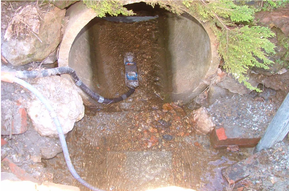
Figure 3. Velocity and depth sensor of flowmeter at the apples site.
