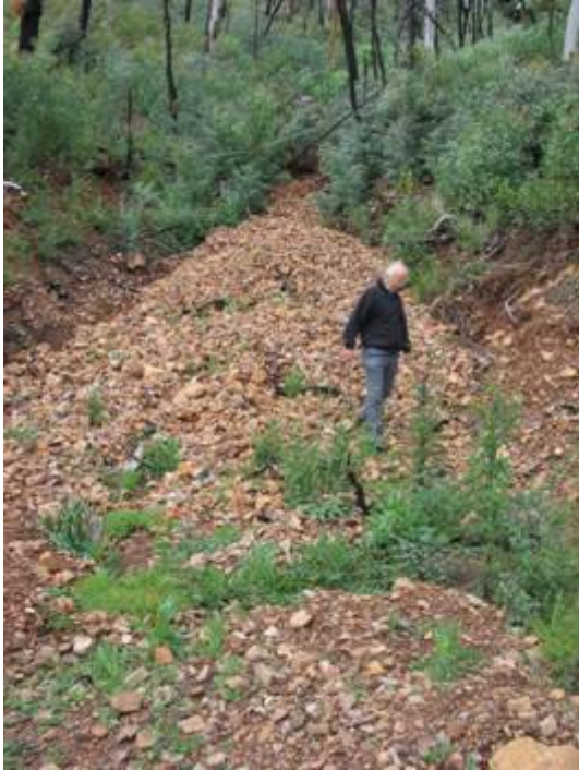
Figure 36. A new gully incision and very coarse material carried by flow from an abandoned road, formed after the 2003 fires hit this native forest in an ACT water supply catchment.
