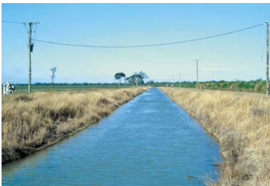
Figure 20. Irrigation water supply channel in Queensland.
