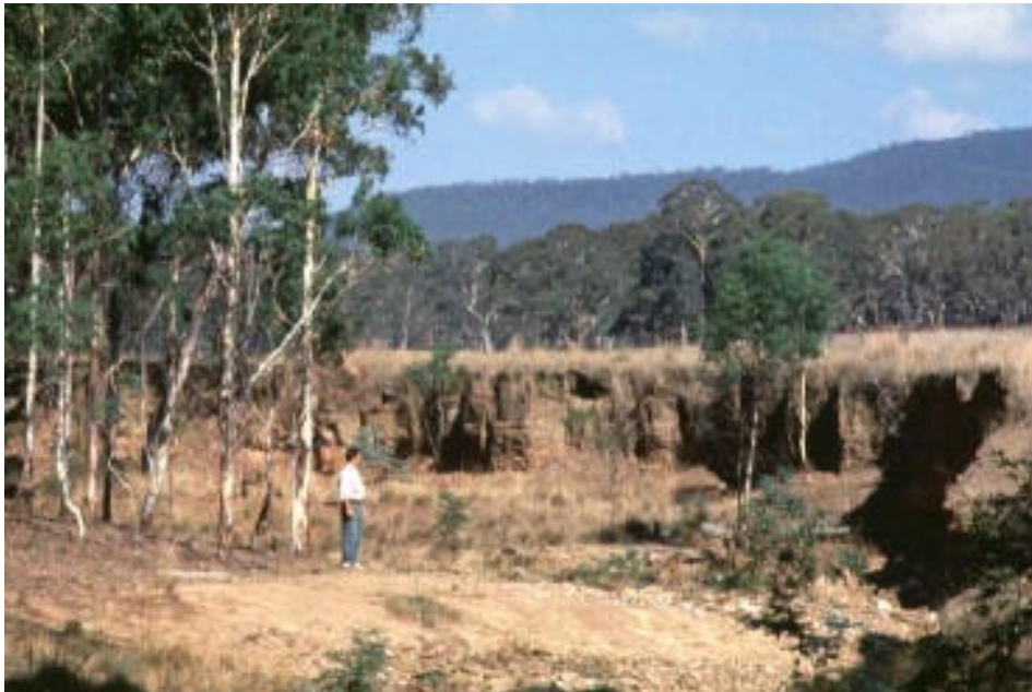
Figure 9.1: Photograph of channel collapse in Molonglo catchment
