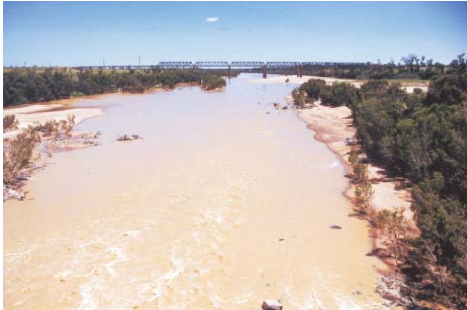
Photo 2: The Burdekin River at the Flinders Highway showing suspended load carried in the water and bedload deposits of sand and gravel.
