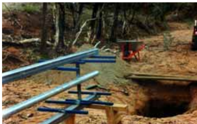
Figure 3.9: Frame with “keys” ready to be concreted into place.
