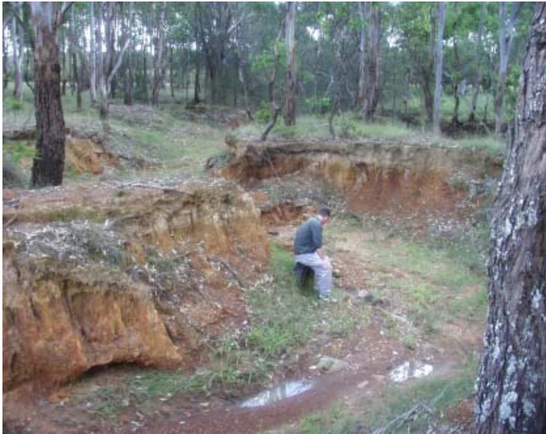
Figure 13. Erosion of Second Pond Creek tributary.
