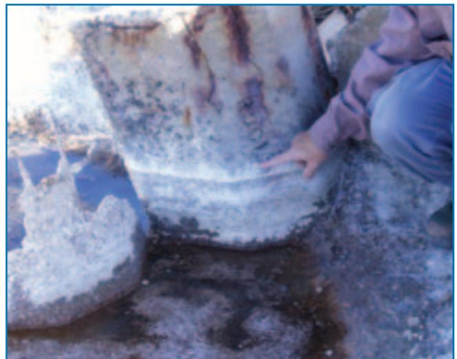
**Figure 3a** Concrete pipe corroded by action of acid sulfate soils
