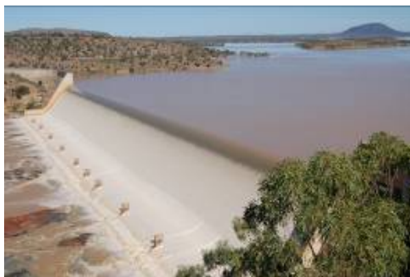
Burdekin Falls Dam – 4 July 2007
