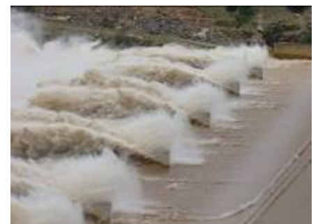
Burdekin Falls Dam Spillway (Photo courtesy of SunWater)
